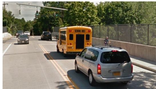
Exhibit 4: Nine bridges over I-95 provide important multi-modal community connections (Weaver St. bridge).
