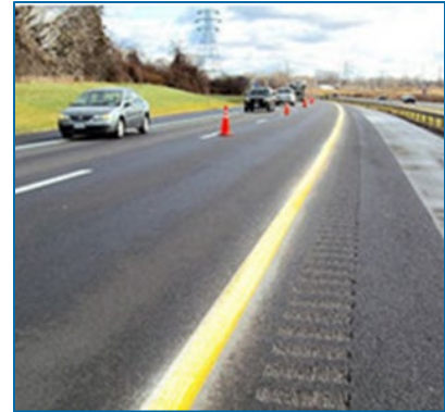
Exhibit 11: Recess Triple Drop pavement markings
